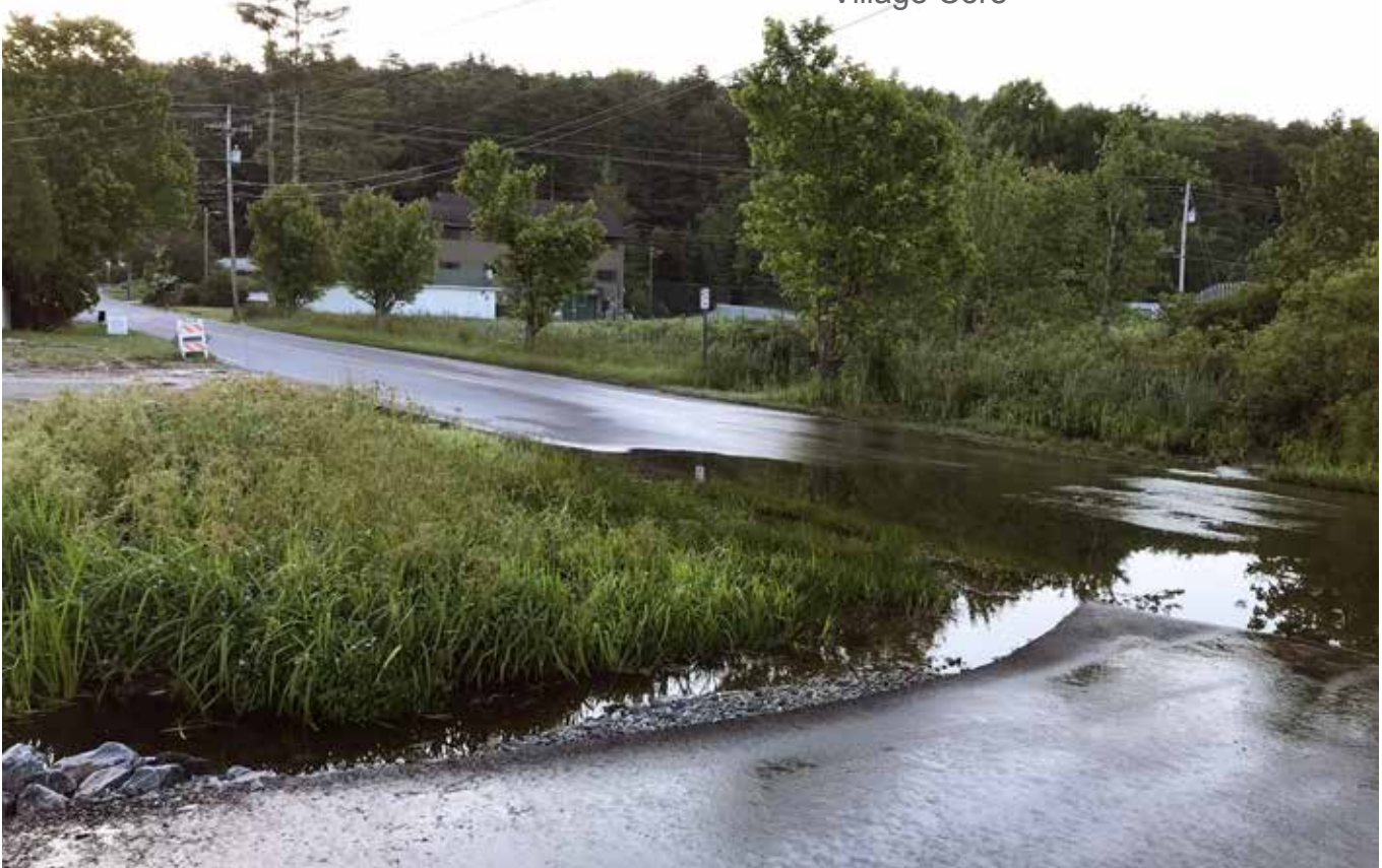
Poor drainage along Frank Allen Road results in a perpetual flow of ground and stormwater. This issue presents a safety hazard and is a significant barrier to walking
