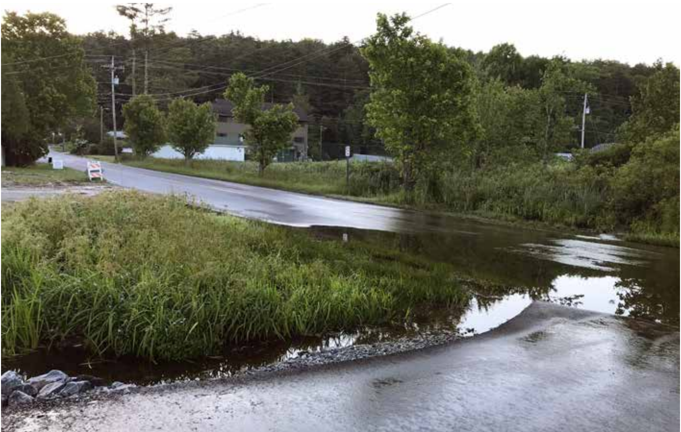
Poor drainage along Allen Road results in a perpetual flow of ground and stormwater. This issue presents a safety hazard and is a significant barrier to walking
