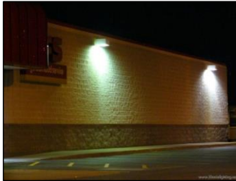
Figure 6.2. Building lighting directed downward
