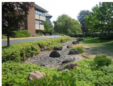
Figure 5. SEQ Figure 1* ARABIC 1 1 Example of vegetated bioswale that catches and filters runoff
