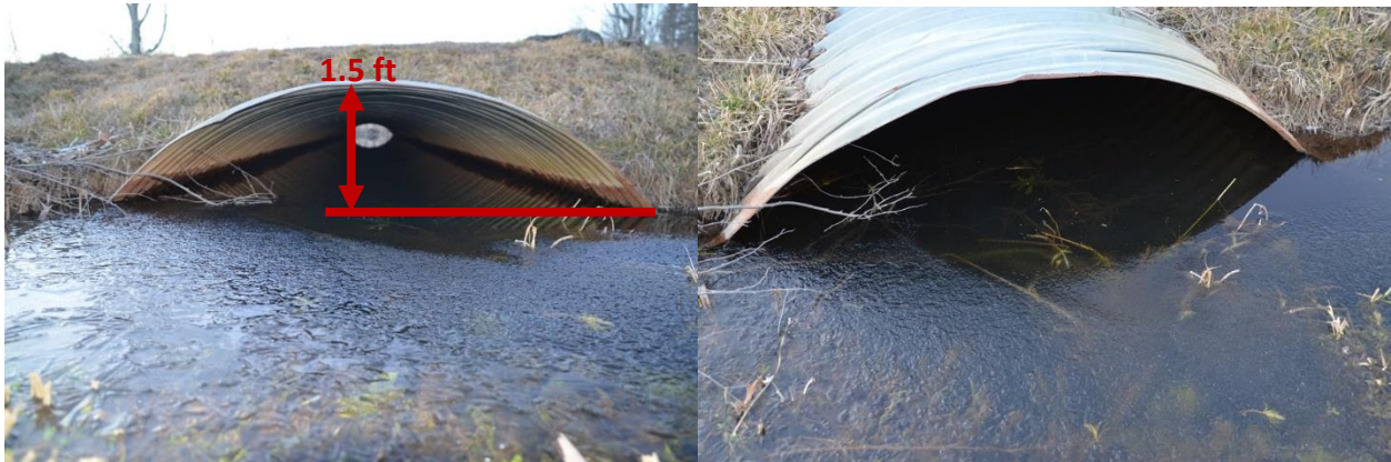
Figure 6. Frank Allen Rd Double Culverts (one culvert from two different angles). For a sense of scale, the culverts are approximately five feet in height. In addition to the high water level, there were many aquatic plants growing near the culvert inlets.
