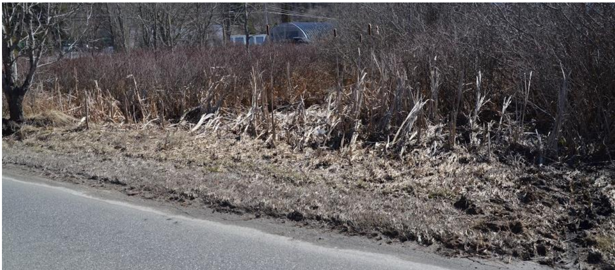
Figure 9. Evidence of Overtopping of Frank Allen Rd. Flatted plant vegetation as evidence of past high water flow conditions. Photo taken on Frank Allen Rd, facing southeast.
