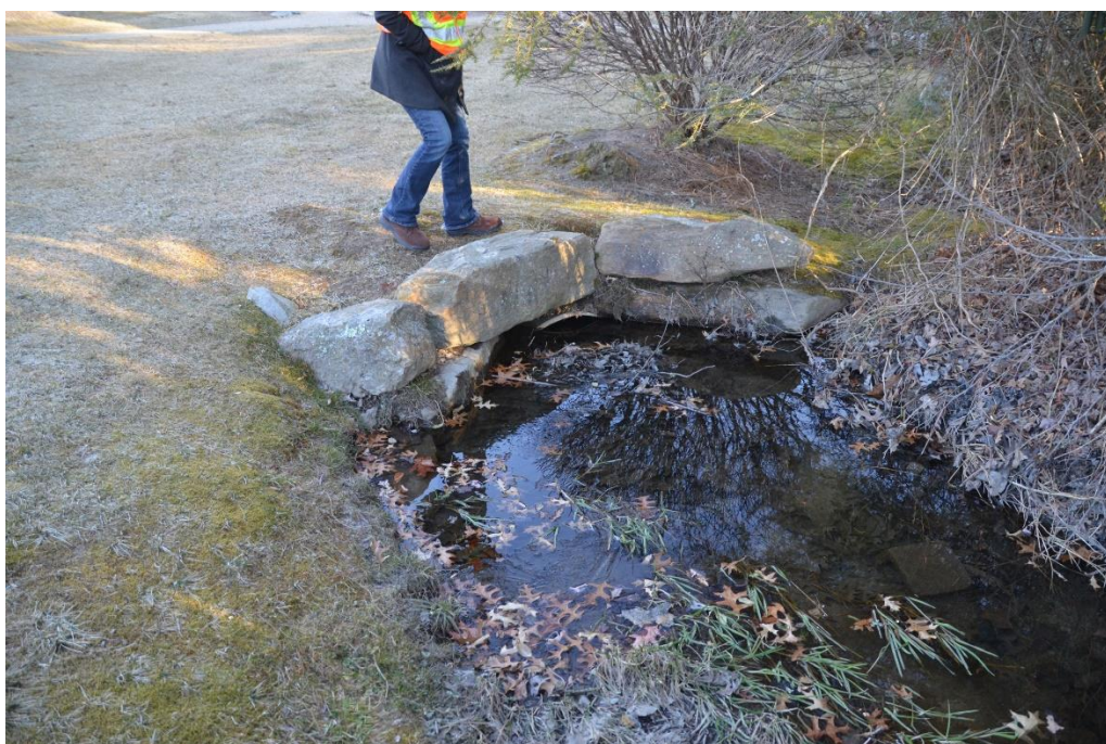
Figure 15. Mouth of culvert connecting Ditch 1 and Ditch 2, after it branches from Ditch 1.
