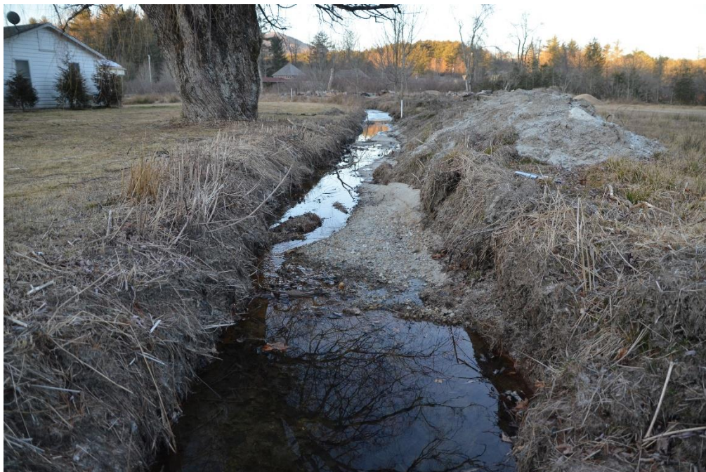
Figure 14. Ditch 3, along with its large amount of sediment deposition
