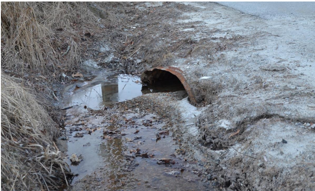
Figure 20. Inlet of culvert 3, with heavy sedimentation.
