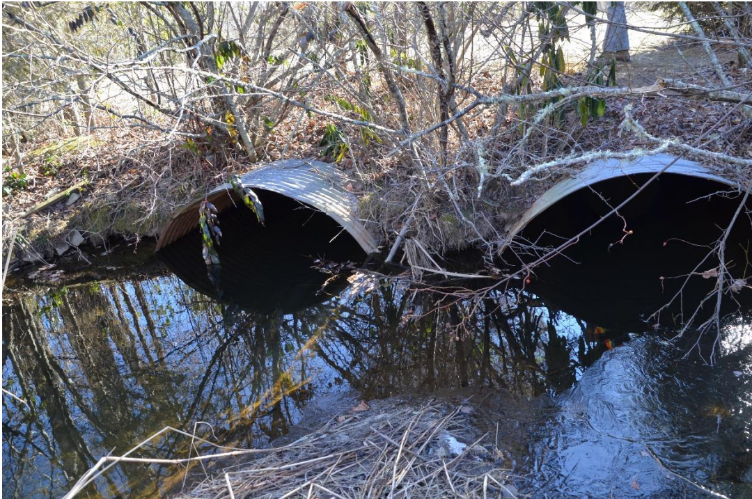
Figure 21. Culvert Set 2 connecting east-side water into Cashiers Creek.
