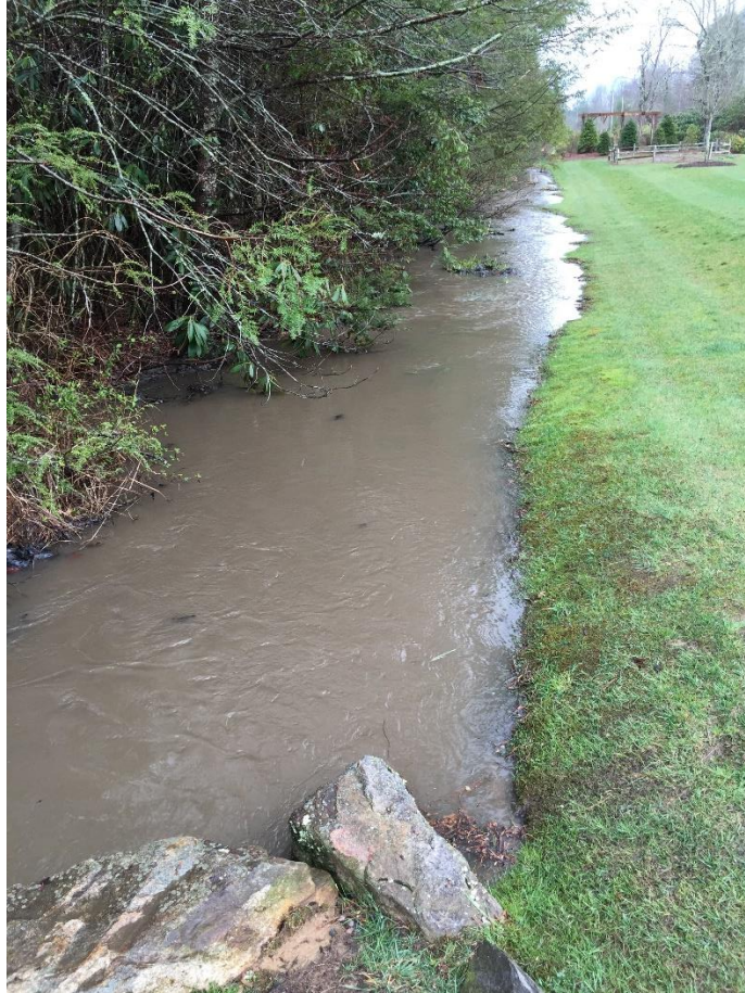
Figure 17. Ditch 2, view is facing downstream towards Cashiers Creek
