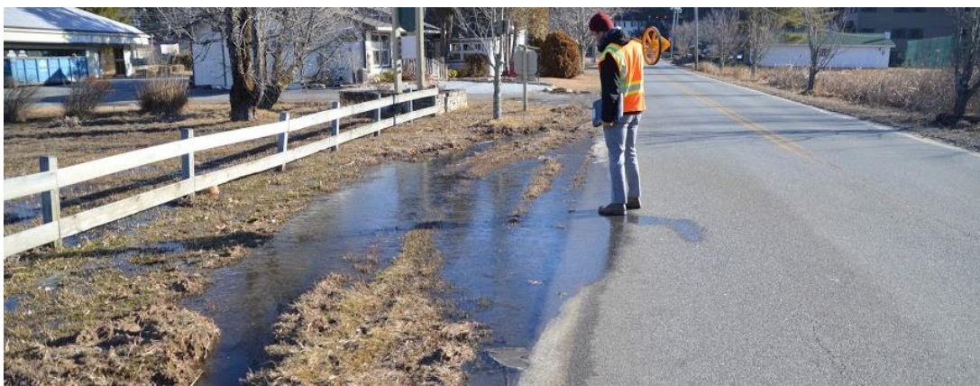
Figure 7. Ponding Along Frank Allen Rd. About 150 ft east of the Frank Allen Rd culverts, the ponding water surface is not connected to the standing water at the culverts.
