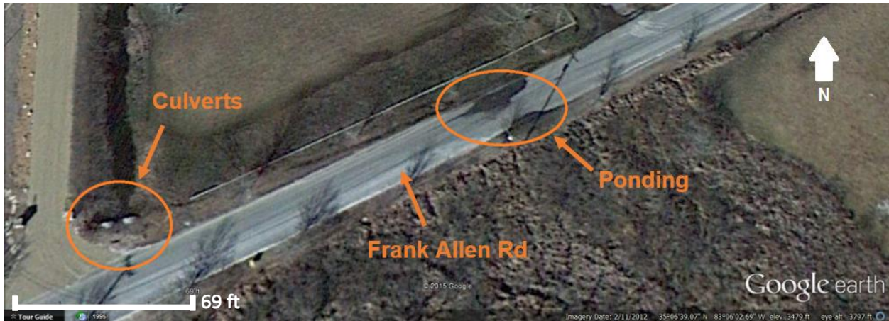
Figure 8. 2012 Frank Allen Rd Ponding. Google Earth image showing ponding along Frank Allen Rd in relation to the Frank Allen Rd culverts. Scale bar is located in bottom left.
