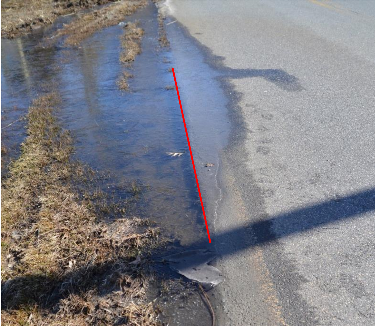
Figure 40. Frank Allen Rd Road Shoulder Material Scour highlighted by the red line, approximately 20 feet in length. Scoured area appears as shadow to the left of the red line.
