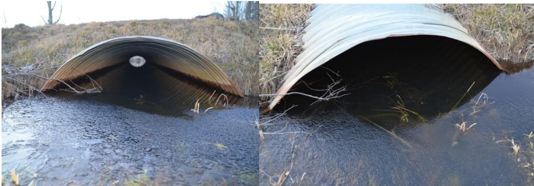
Figure 22. Culvert Set 1 right below Frank Allen Rd.
