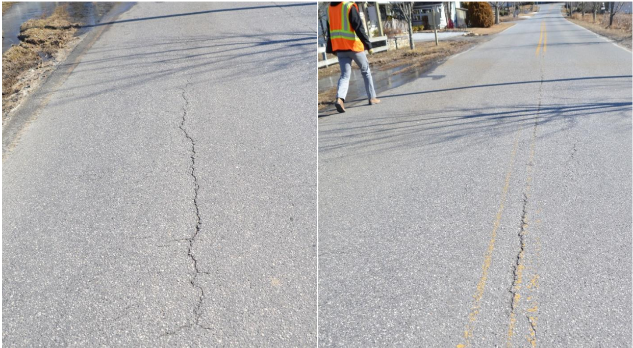
Figure 38. Frank Allen Rd Longitudinal Cracks. Left photo shows a crack in the center of the lane, outside of the wheel-path. Right photo shows a crack along the lane striping, outside of the wheel-path. Average crack width < 0.5 inches.
